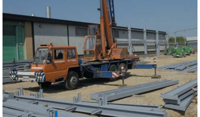
The factory extension is well on its way to be completed.
